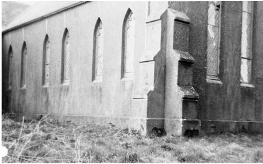
Pillaton Chapel SW Buttress (ca 1970)
