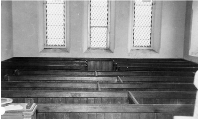
Pillaton Chapel SE Windows (ca 1970)
