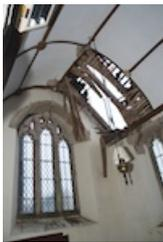
Work has started on making the church safe by removing some of the large granite blocks that were still perched on the roof and covering up the holes there to prevent rain and snow from coming in.
