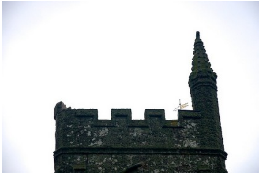
Close up of the tower
